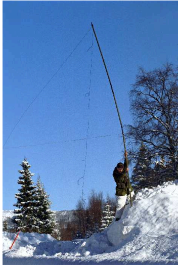
Figure: 5.18 Erecting field communications lines
