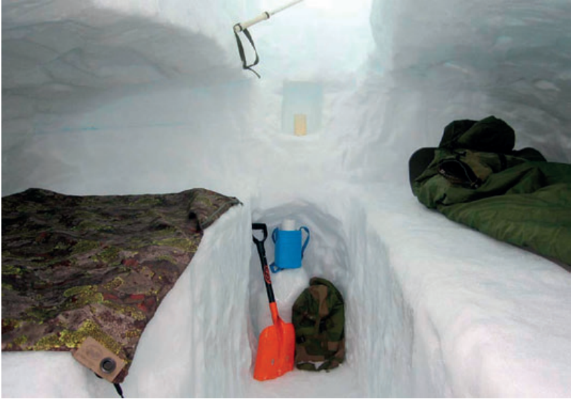
Figure 55 - Fitting up a flat pit
