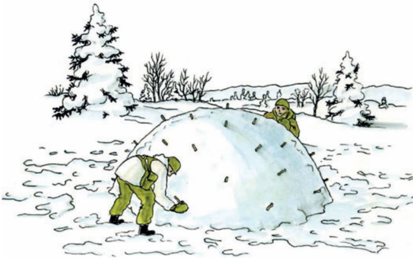
Figure 52 - Inserting sticks to mark the thickness of the igloo
