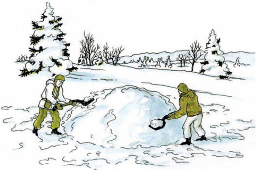
Figure 51 - Building up the snow mound for the igloo
