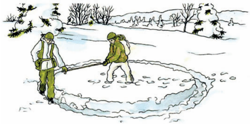
Figure 50 - Stepping down the circumference of the igloo
